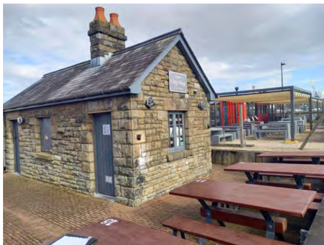
Photograph 5: View of one of the buildings on site (B13) looking east.
