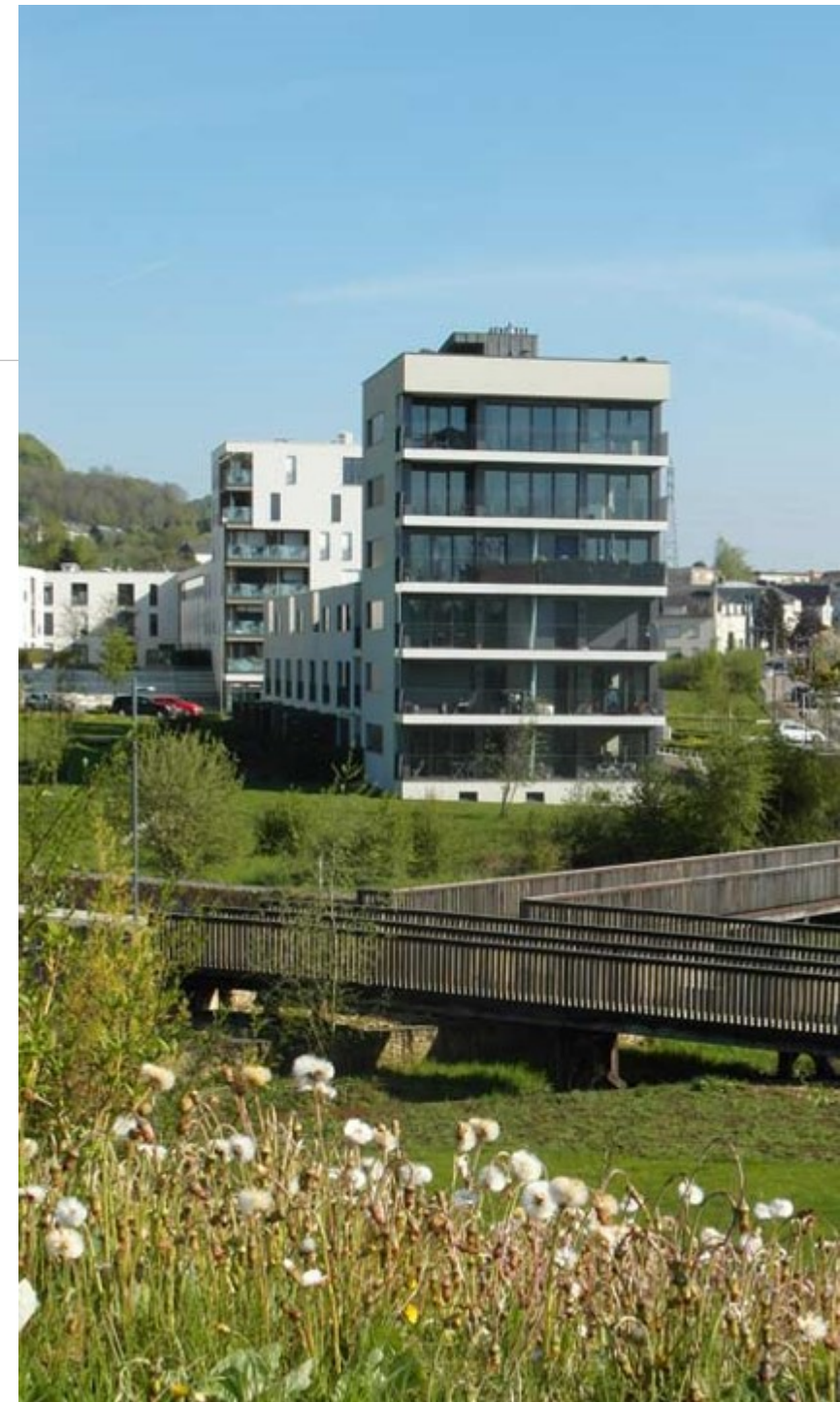
Parc Um Belval/ Water-retention Boulevard, Luxembourg
