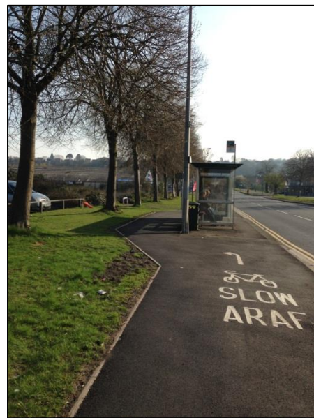
Footway / Cycleway – Penarth Road
