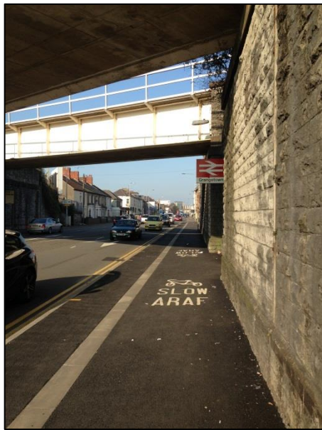
Footway / Cycleway – Grangetown
