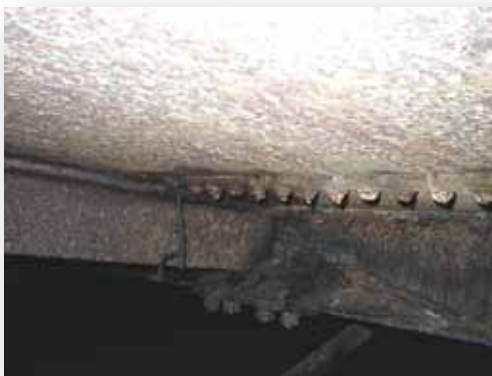
Photograph 4 Internal structure (c.2000)
