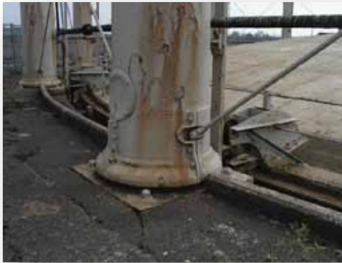
Photograph 2 Column No. 1 (c.2000)
