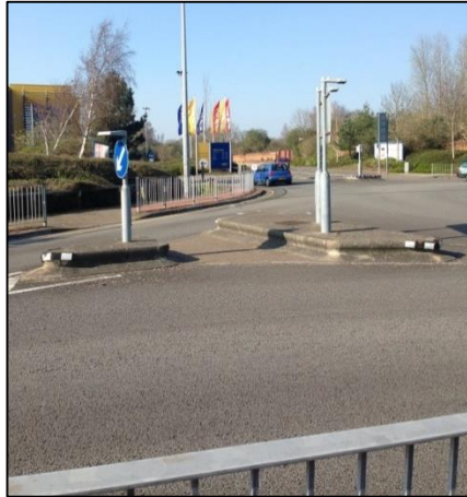
Photograph 1 – Site Access / Ferry Road Rbt
