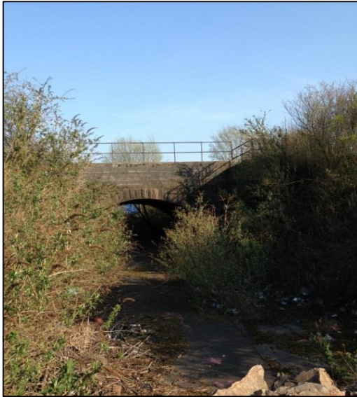
Photograph 15 – Existing Link connecting to Fleet Way
