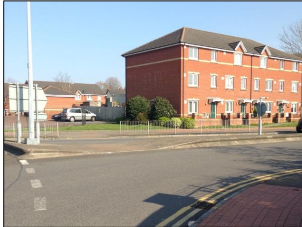
Photograph 2 – Site Access / Ferry Road Roundabout
