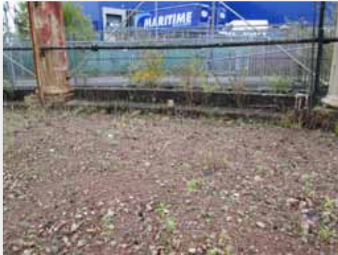
Photograph 7 Tank edging and kerb
