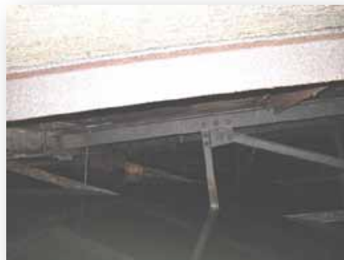
Photograph 5 Internal structure (c.2000)
